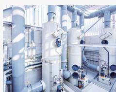
Exhaust air purification systems made of plastic for treating environmentally hazardous exhaust air and gases
