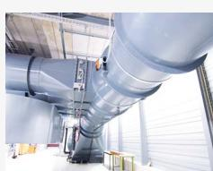
Ventilation systems made of plastic for efficient routing of corrosive exhaust air and gases
