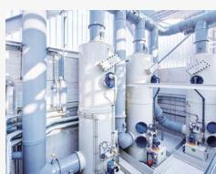
Exhaust air purification systems made of plastic for treating environmentally hazardous exhaust air and gases
