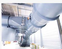
Ventilation systems made of plastic for efficient routing of corrosive exhaust air and gases
